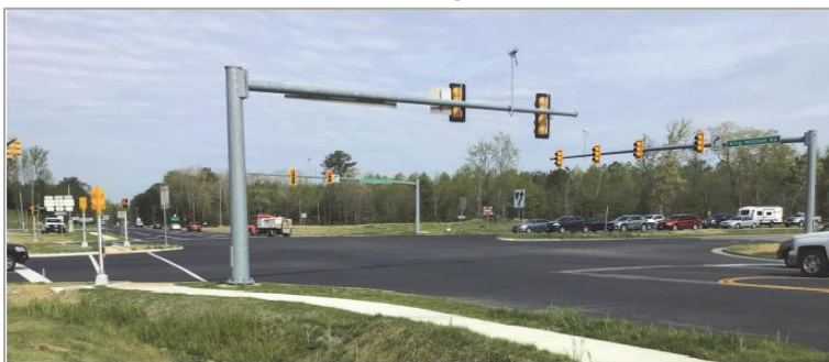
Rt 360 and Rt 30 Intersection Improvements, 2021. VDOT.
