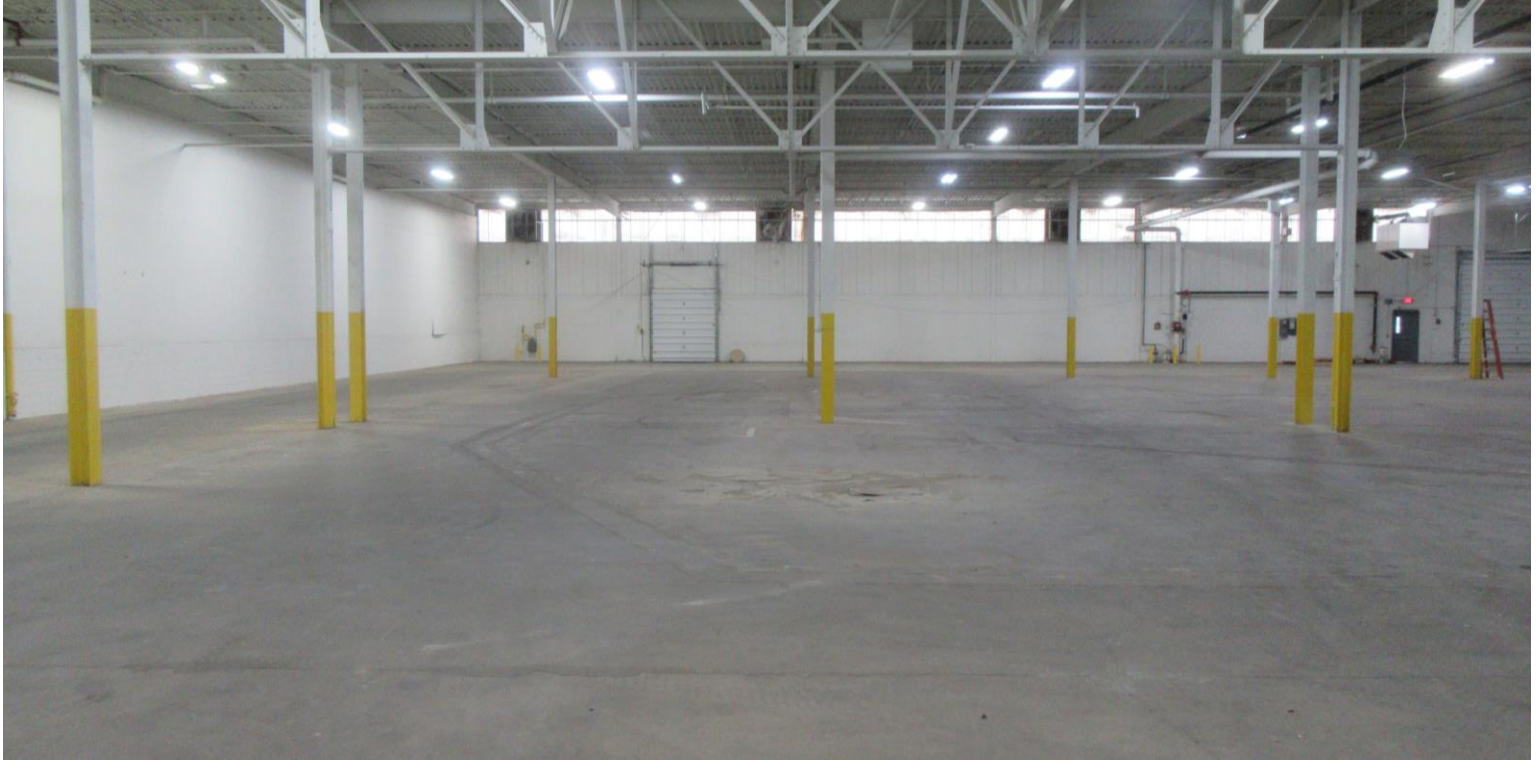
Interior Warehouse View
