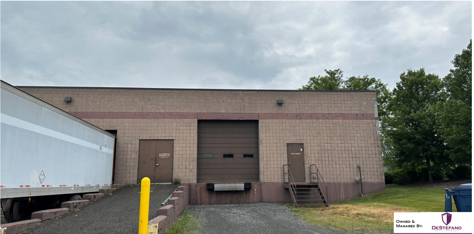
Dock and drive in door
