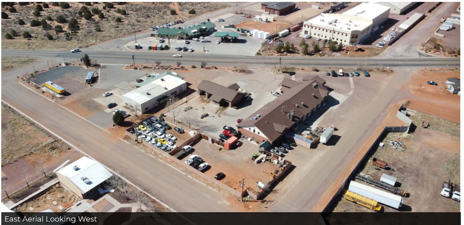
Northwest Aerial Looking Southeast
