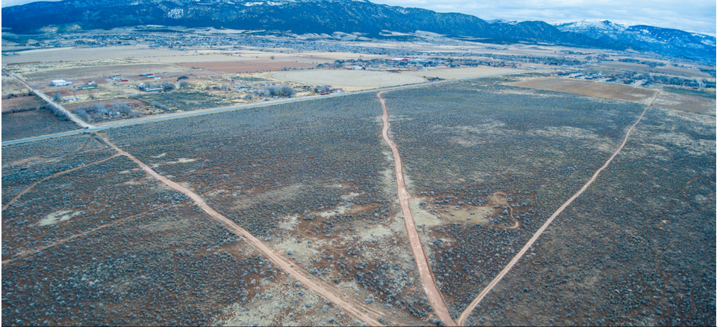
Northwest Aerial Looking Southeast
