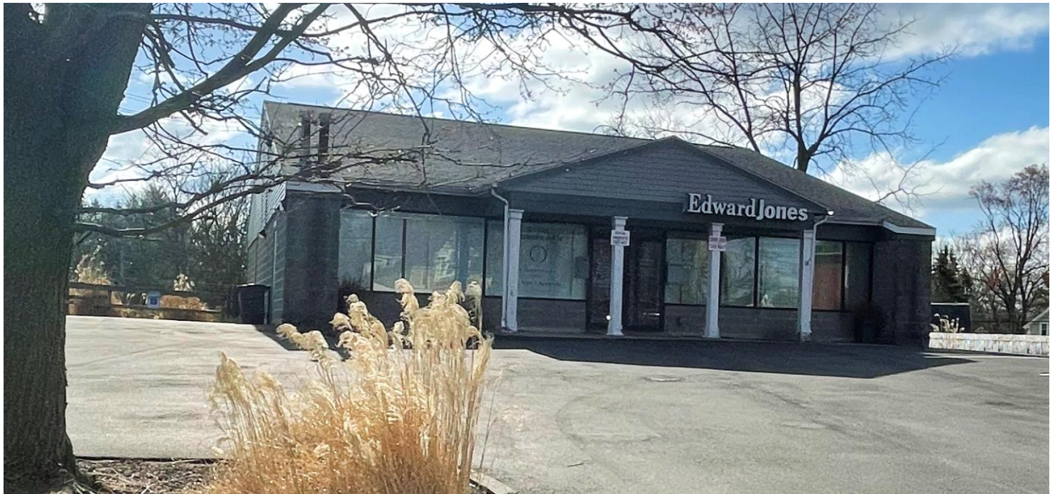
South Main Street Entrance
