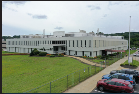
I-290Connector Pre-renovation View
