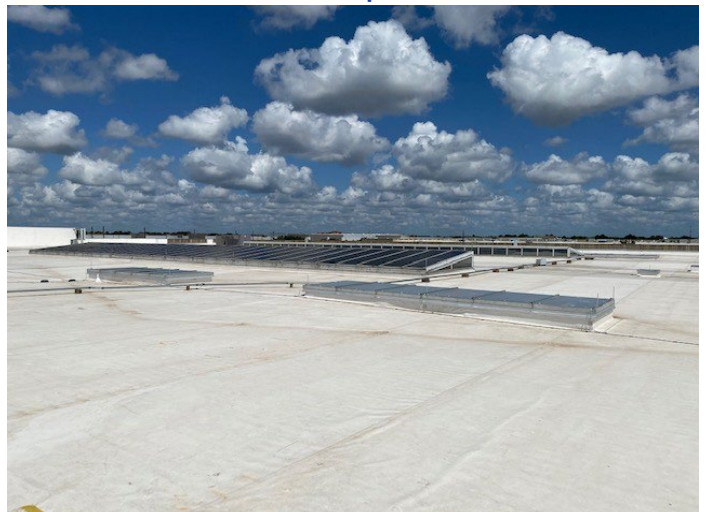
New TPO roof
