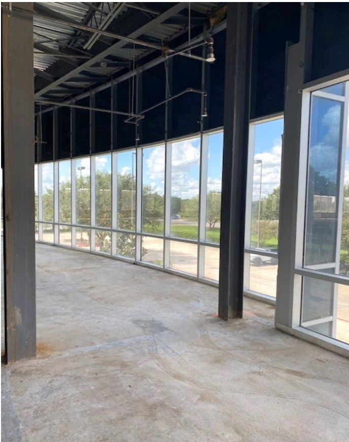
Full-height glass at front of the building
