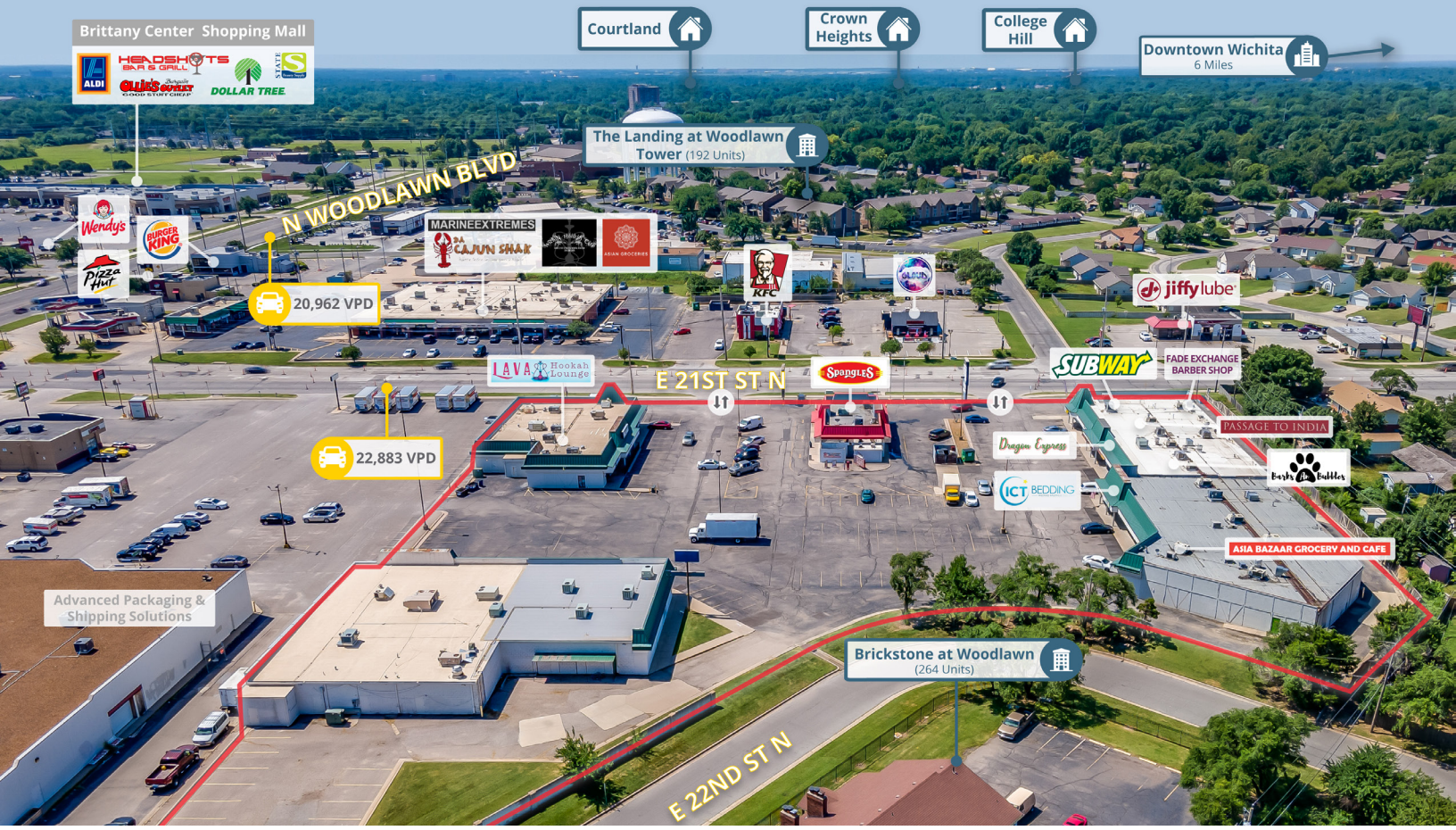
South Facing View
