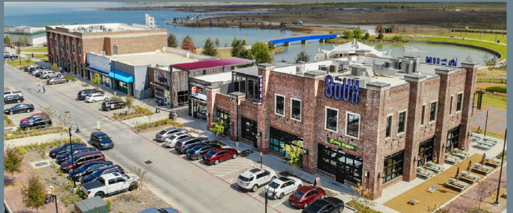
North Building West Elevation
