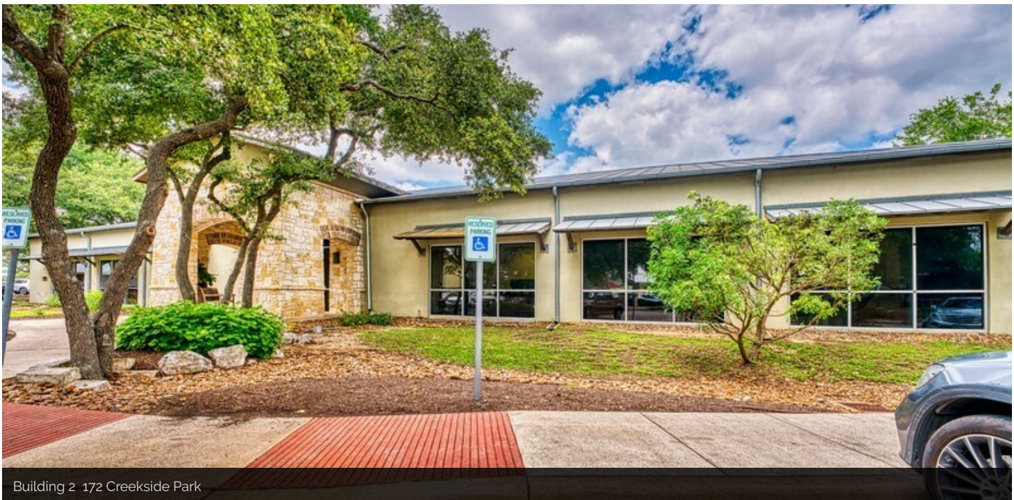
Building 2 172 Creekside Park
