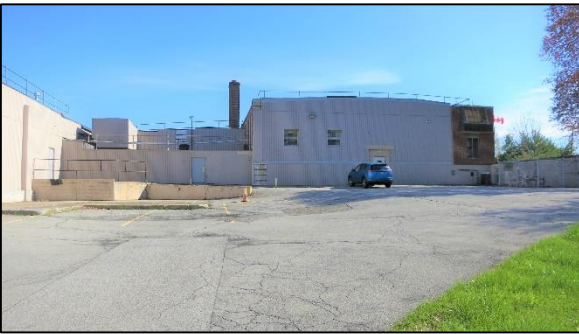
Office Area from South
