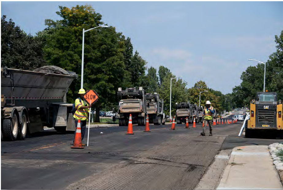
Annual pavement management program underway
