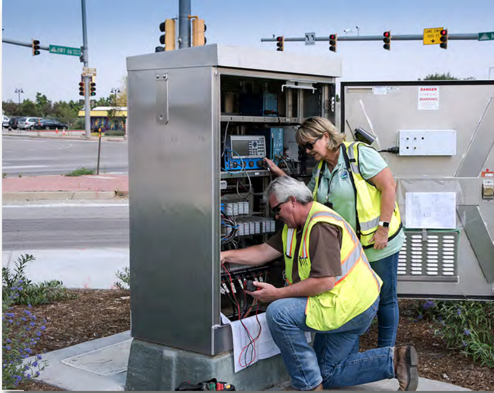
City of Longmont streetlight technicians at work
