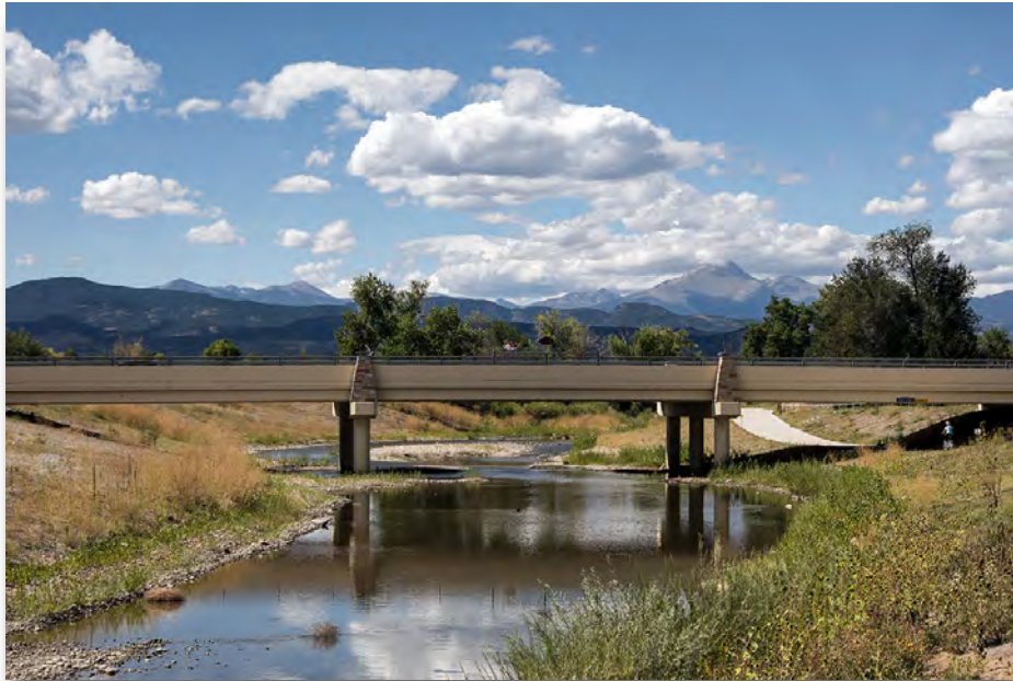
The new Sunset Street Bridge over St. Vrain Creek
