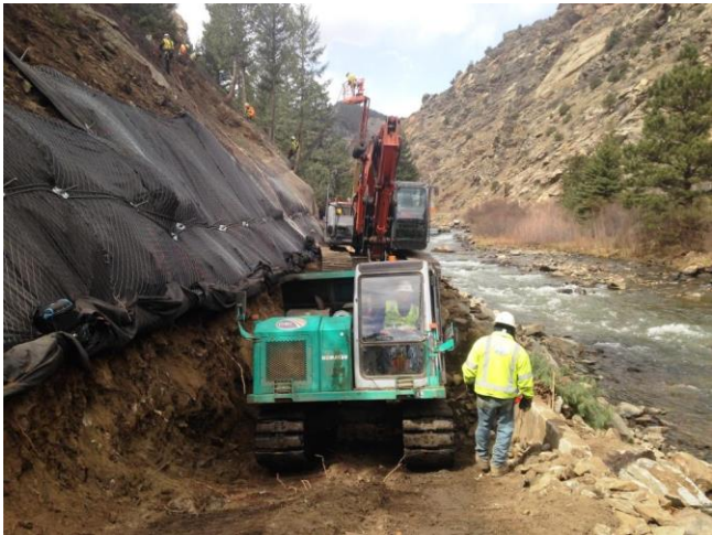
Peaks to Plains Trail Construction, Clear Creek Canyon Park
