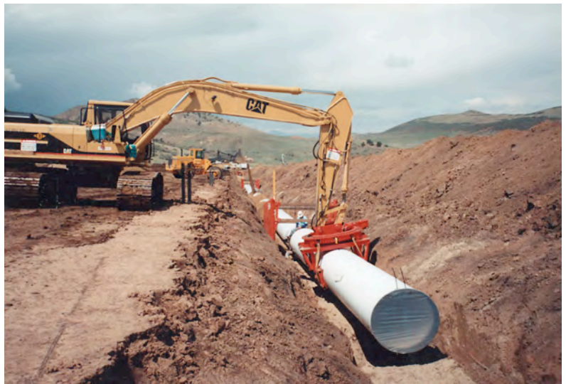
Southern Water Supply Project construction in the 1990's
