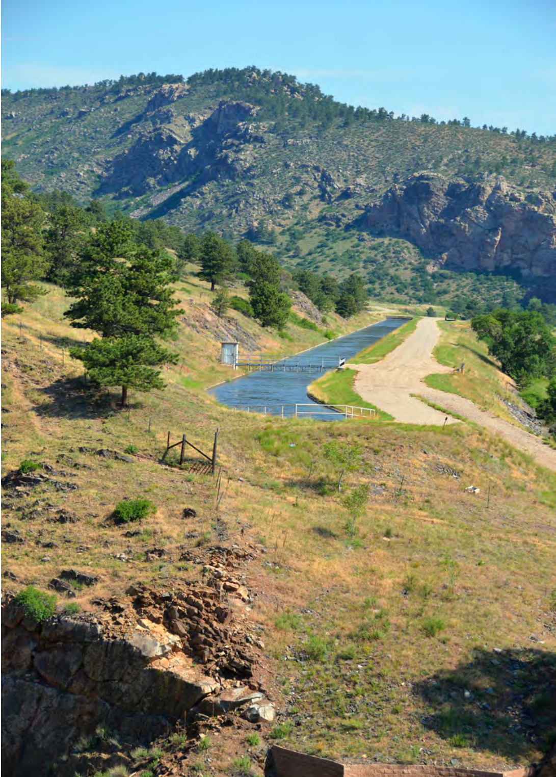
Hansen Feeder Canal
