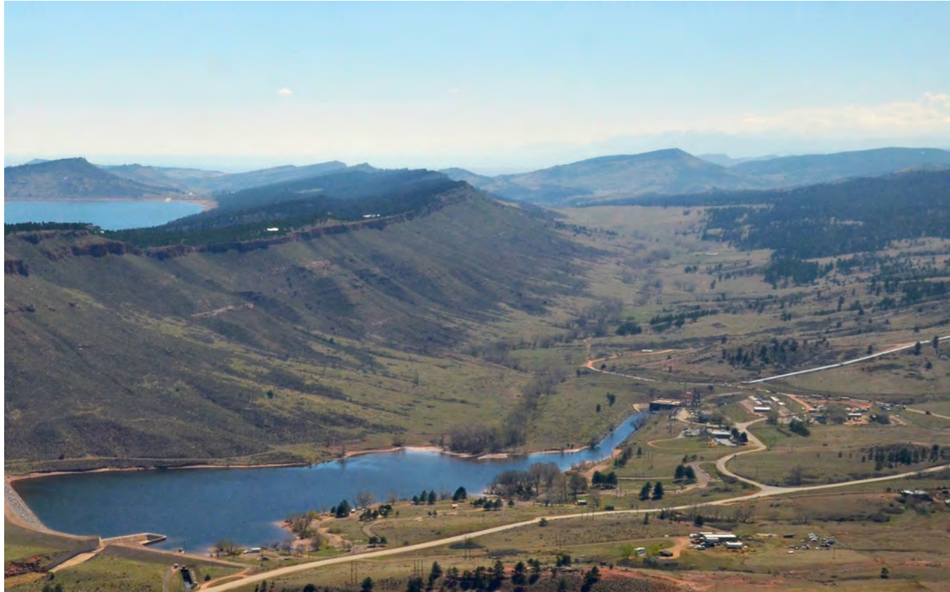
Site of the proposed Chimney Hollow Reservoir, with Flatiron Reservoir in the foreground and Carter Lake to the left
