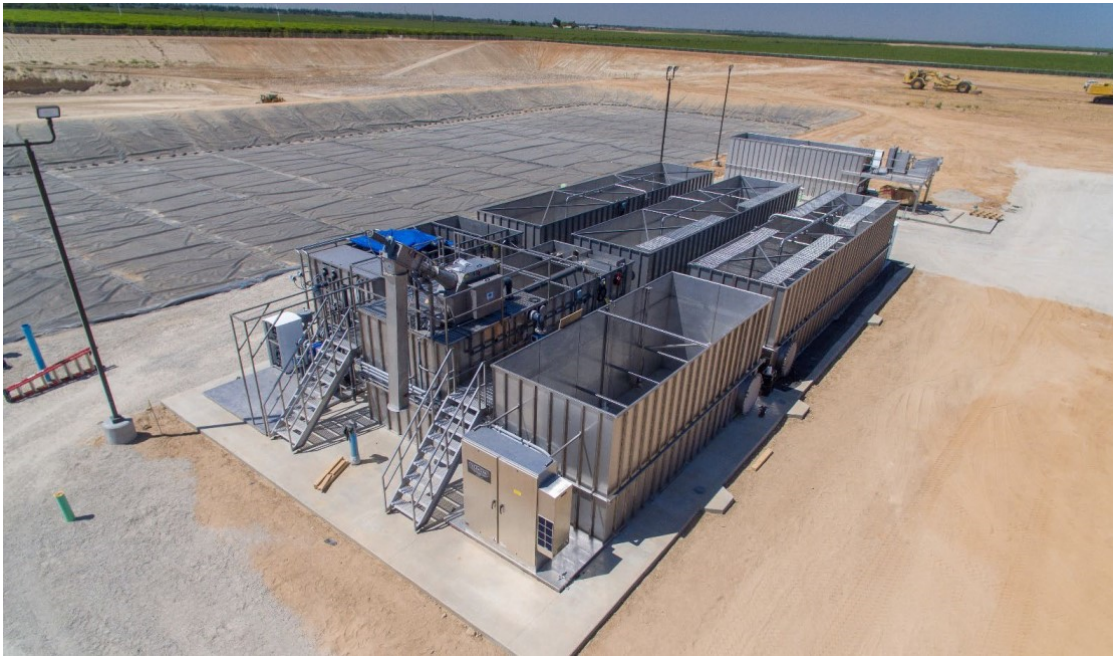
Figure 3-2: Example Packaged MBR
