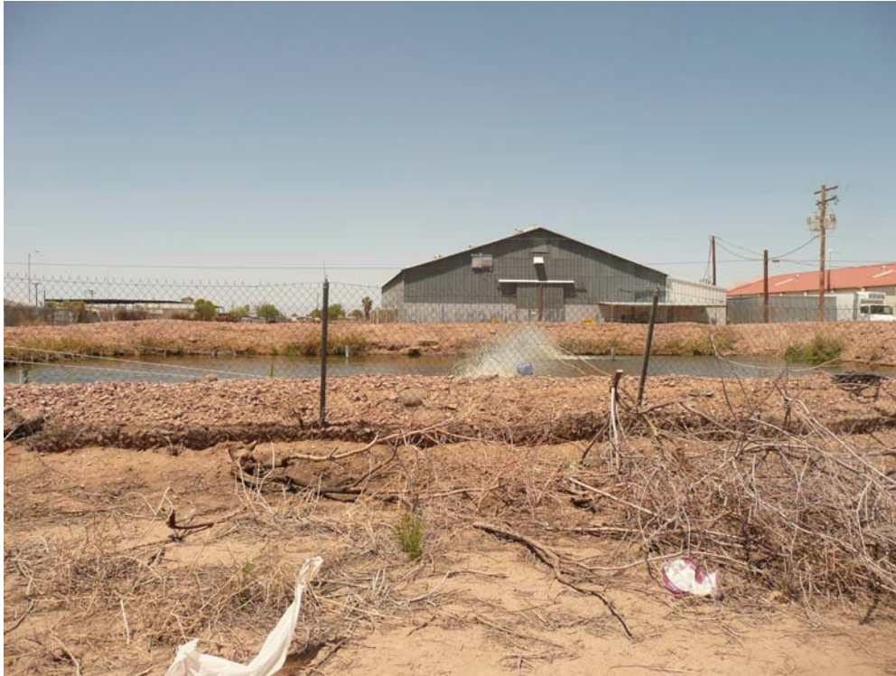
View of aeration pond, view west from northwestern corner of subject site.
