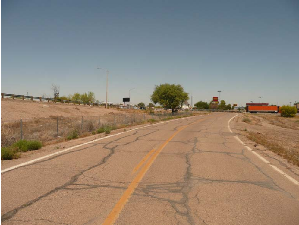
View northwest from northwest corner of subject site.
