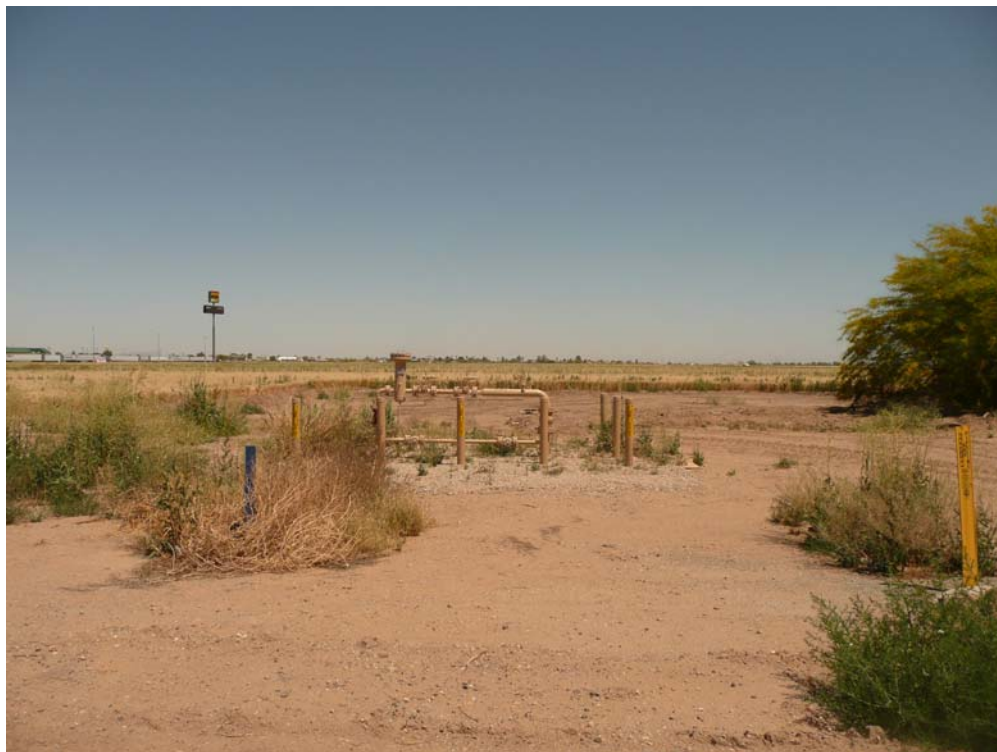
Natural gas connection, view north from Milligan Road of subject site.
