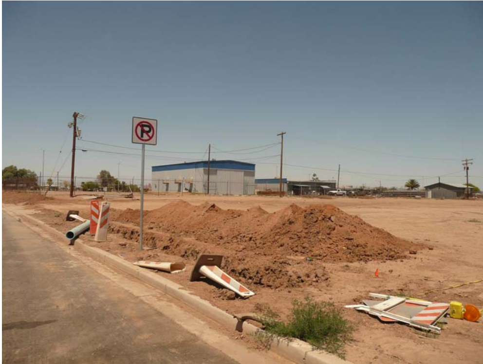
View west from Date Street Sunshine Boulevard.
