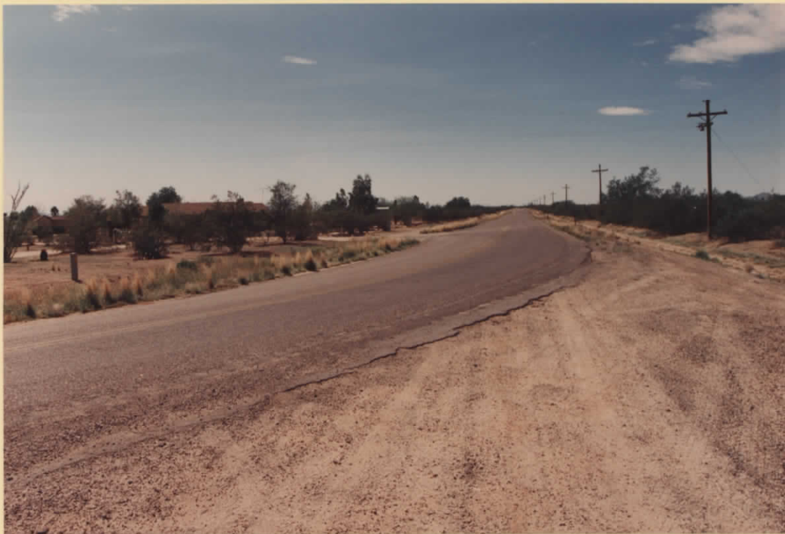
(8) LOOKING WEST ALONG WOODRUFF ROAD FROM SOUTH BORDER OF SITE. (SEE SITE PHOTO KEY)
