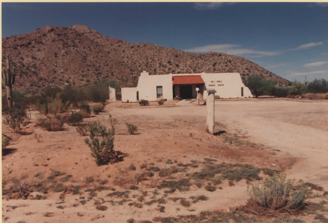
(4) OFF-SITE BUILDING AT SOUTHEAST CORNER OF SITE. (SEE SITE PHOTO KEY)
