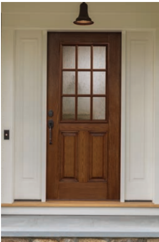
Simulated Divided Light with Textured Glass
