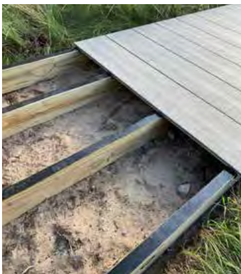
Add joist tape for protection
