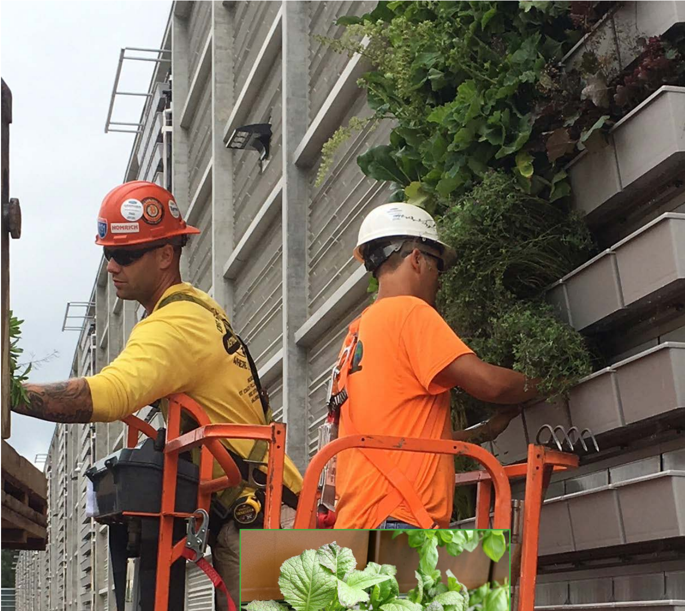
Place planted inserts into the wall planters according to specified design.
