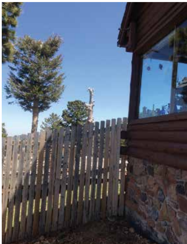
Figure 3.20. Fire could spread directly from this combustible wood fence to the structure; within five feet of structures, fence sections should be noncombustible (Wildland Professional Solutions)
