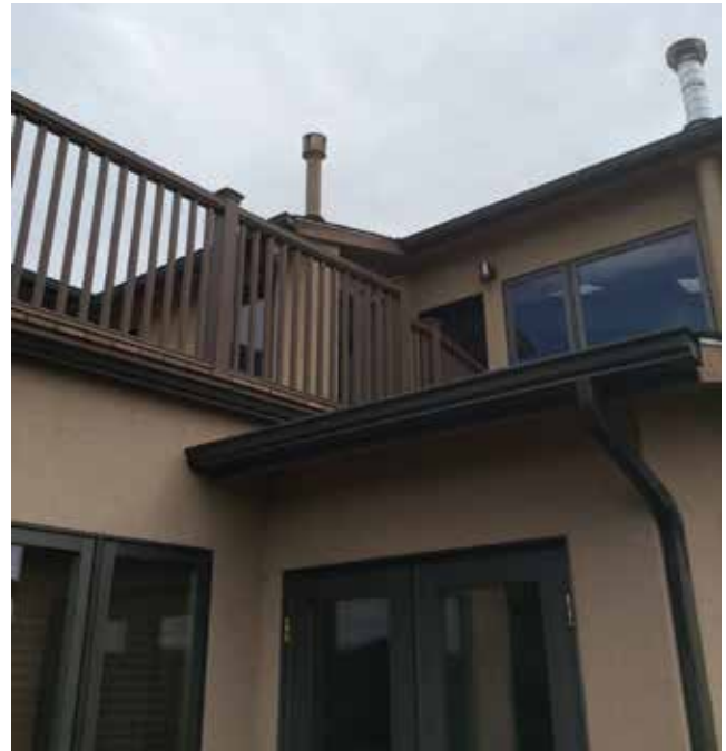
Figure 7.7. Ignition-resistant siding (such as stucco), multipaned or tempered glass windows, noncombustible gutters, enclosed eaves, and other features are typical requirements in building codes that address the WUI (Wildfire Planning International)
