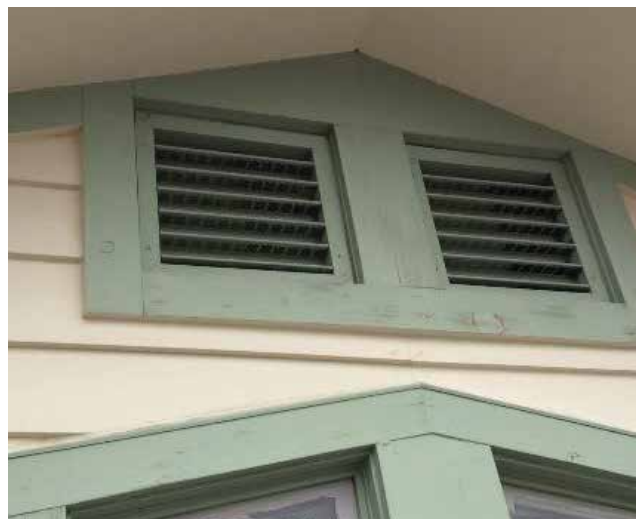
Figure 3.16. These gable attic vents have openings that are smaller than one-eighth inch and are therefore effective at mitigating ember entry into the attic space (Wildland Professional Solutions)
