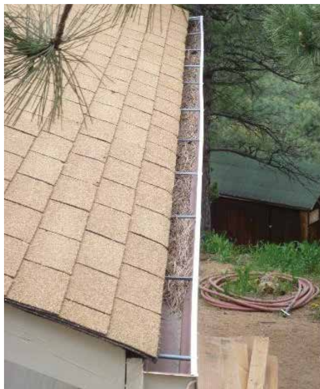
Figure 3.17. Though this noncombustible gutter will not melt, the combustible debris within it could lead to ignition of any unprotected roof sheathing under the fire-rated roof covering (Wildland Professional Solutions)
