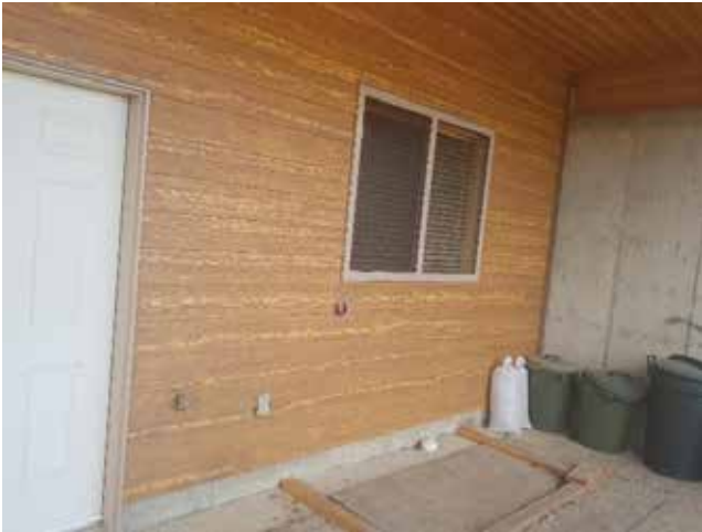
Figure 3.18. The bottom six inches of this exterior wall is constructed of noncombustible concrete, which in this case is part of the structure's foundation (Wildland Professional Solutions)
