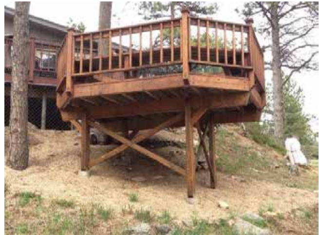
Figure 3.19. A heavy timber deck over a noncombustible surface that extends five feet from the perimeter of the deck (Wildland Professional Solutions)
