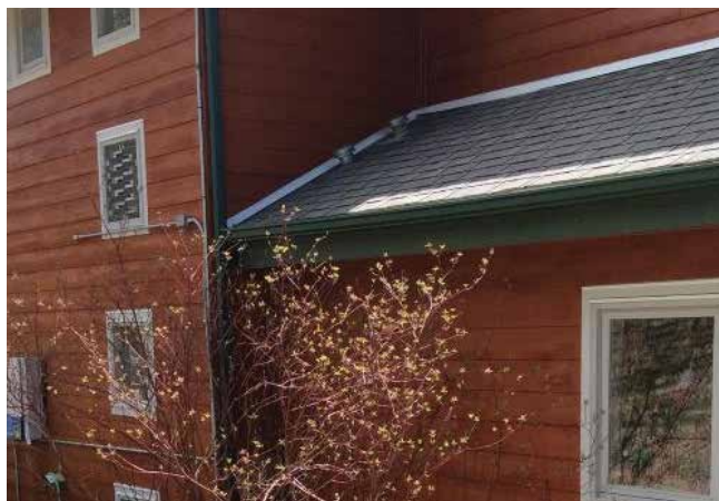
Figure 3.15. An example of a complex roof design in which combustible siding extending above the roof line is protected with two inches of noncombustible flashing (Wildland Professional Solutions)
