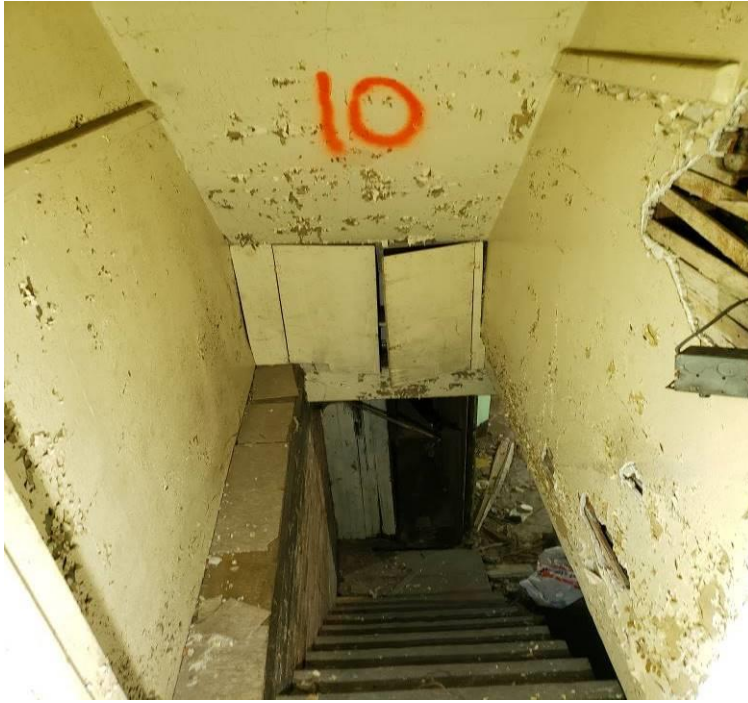
View of FS-10 1 st floor stairs to basement
