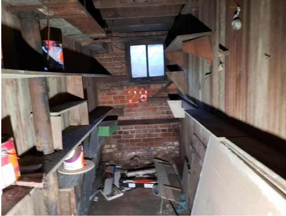
View of FS-28 (basement)
