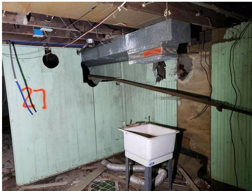
View of FS-27 (basement)
