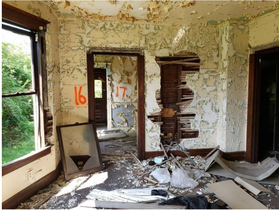
View of FS-16 (2 nd floor unit)
