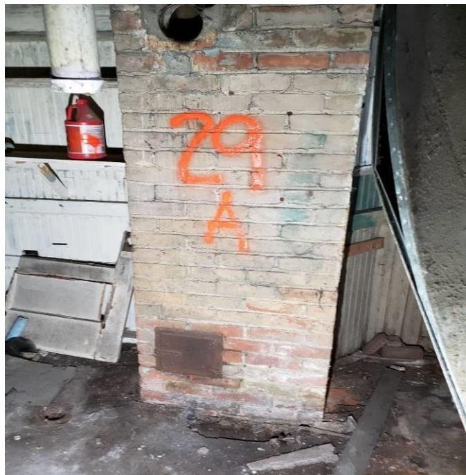
View of FS-29 (chimney stack A)
