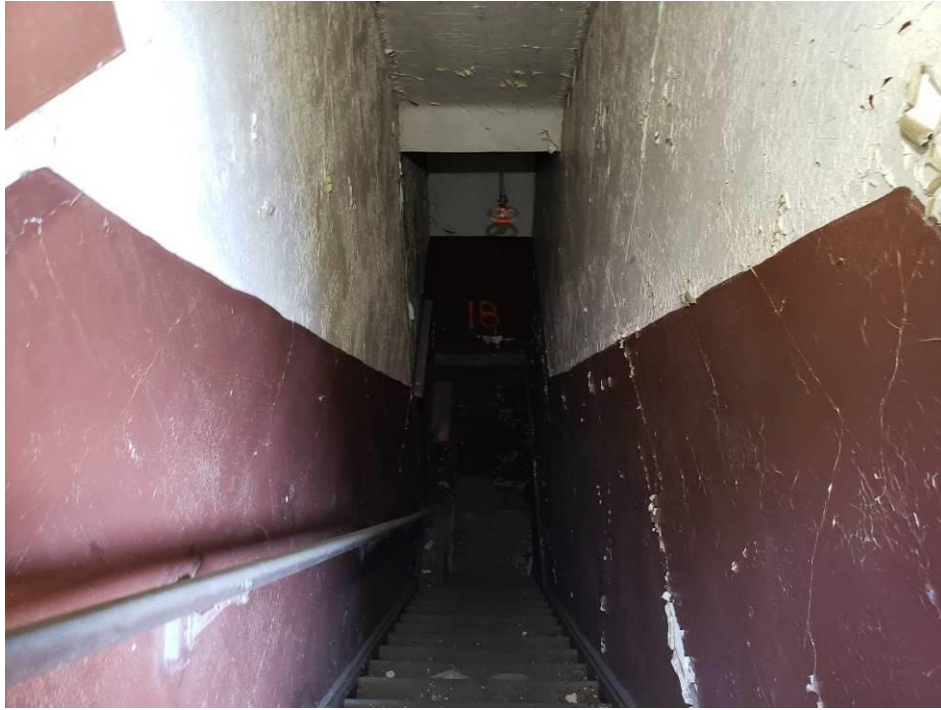
View of FS-18 (2 nd floor unit) – stairs to basement area
