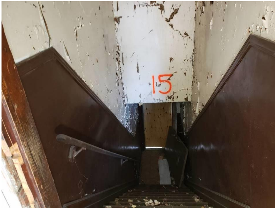
View of FS-15 stairs to 2 nd floor unit
