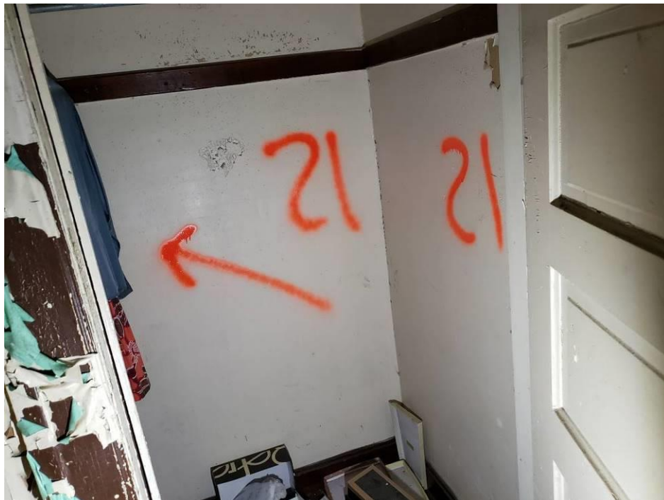
View of FS-21 (2 nd floor unit) – stairs to attic
