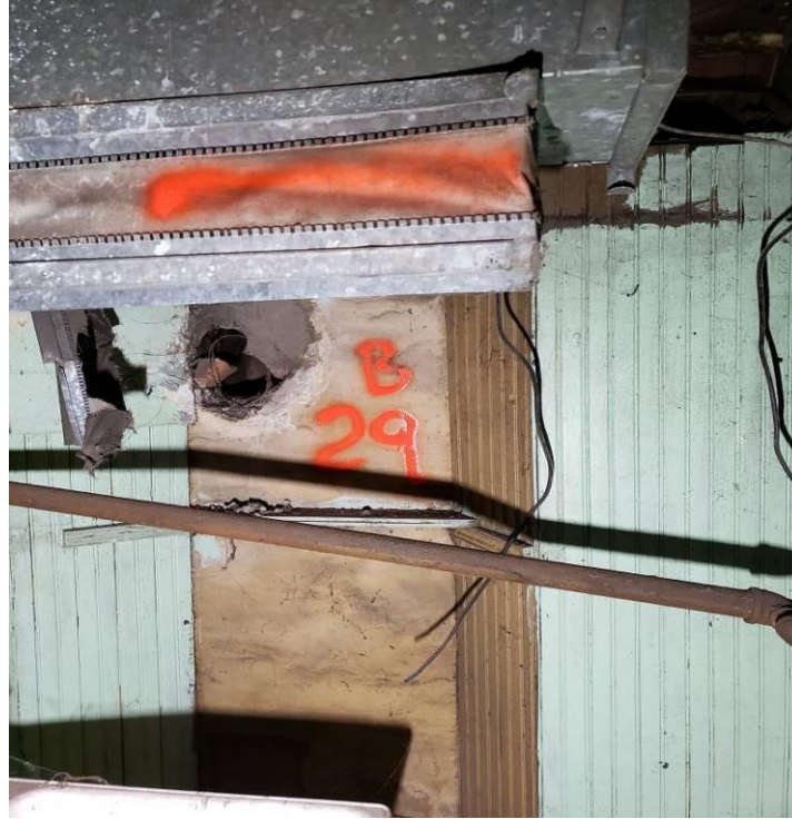
View of FS-29 ( chimney stack B)
