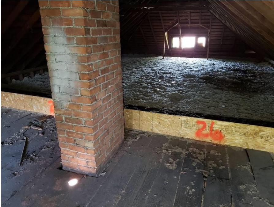
View of FS-26 (attic)
