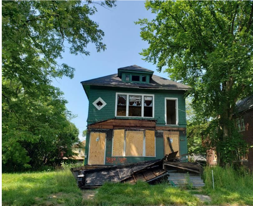
Street view of the house located at 3889 / 3891 St. Clair Street (EA-1) and roof (EA-5)
