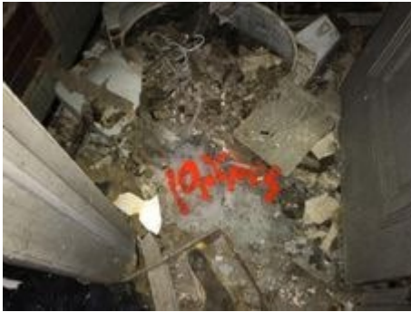
AS 19-1 Floor Mortar
