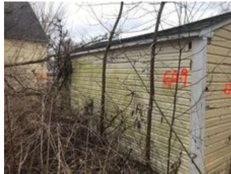
EA-9: Right Side of Garage
