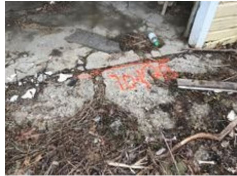
AS 10-1 Driveway Expansion Joint
