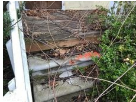
AS 5-1 Porch Concrete
