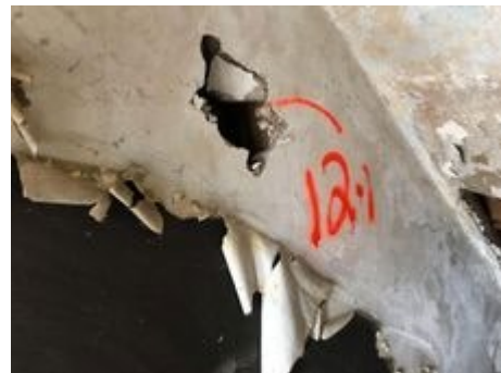
AS 12-1 Plaster On Backerboard
