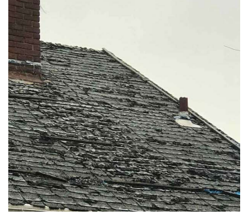
Deteriorated shingles
