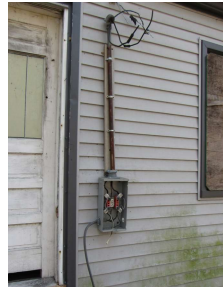
Exposed conductor
