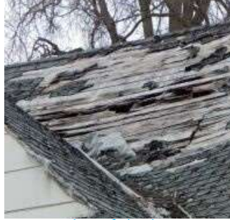
Exposed roof deck
