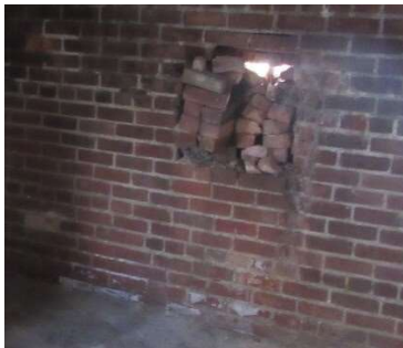
Open brick foundation
