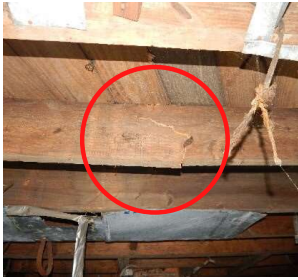
Cracked joist
