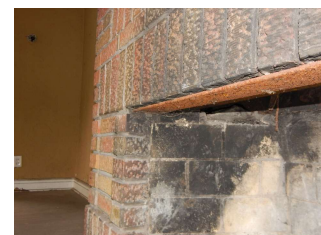
Damaged firebrick
