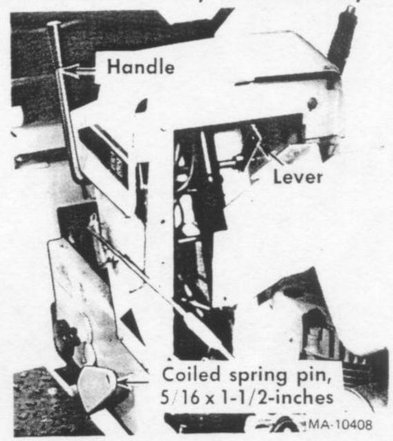
STEP 8. ATTACHING CONTROL VALVE TO PEDESTAL,
