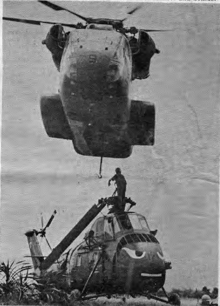
TEAM EFFORT—A CH-53 Sea Stallion from Marine Heavy Helicopter Squadron-463 prepares to lift a downed UH-34 from a landing zone. The lift was successful despite enemy fire directed at the CH-53 and Cpl. Claude H. Anderson, 19, (Atlanta, Ga.) of the recovery team, waiting to make the hook up. (Photo by: Sgt. Rich Groscoft)
