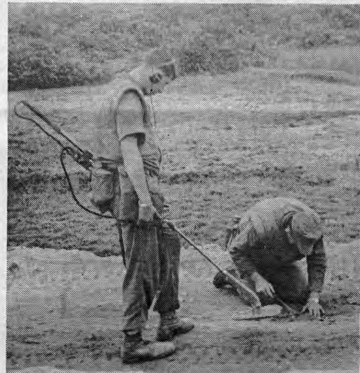
EASY DOES IT—Marine engineers probe for Viet Cong mines on Highway 1, the longest convoy route in Vietnam.
