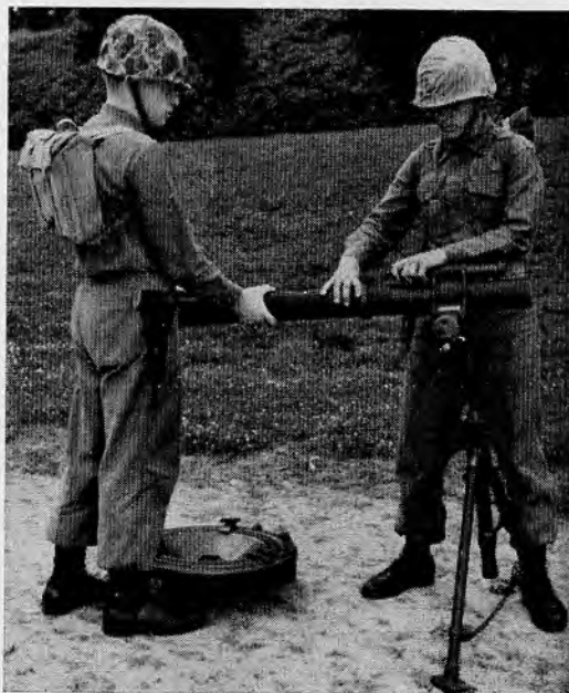
Fig. 30.11 Inserting the barrel into the yoke assembly.
