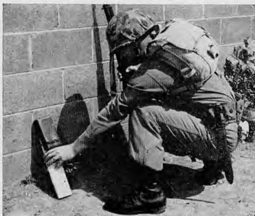
18.6 This Marine is about to "mouse hole" a building with a pole charge.
