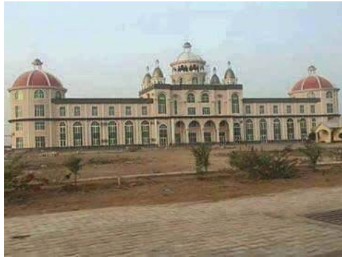
North West University, Kano Nigeria
