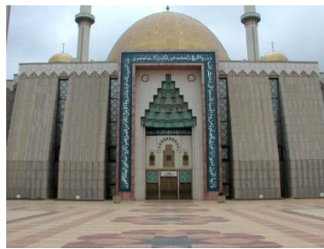
Abuja National Mosque, 1980 (Mosque, 2017)
