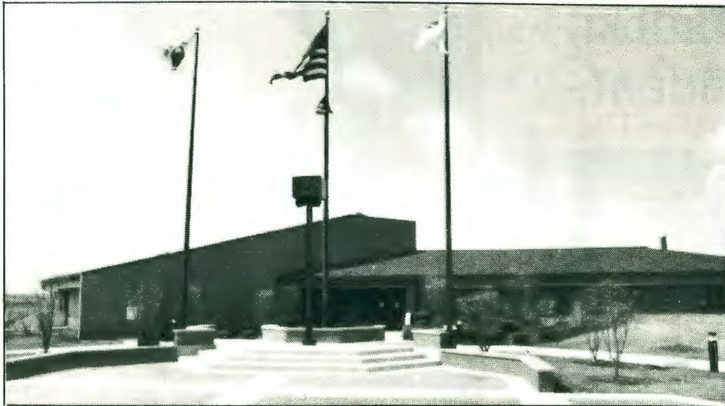
Tinley Park Village Hall, 16250 Oak Park Ave.
