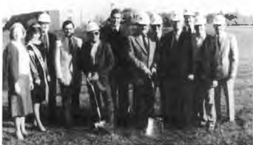
Original Ground Breaking FALL 1986
