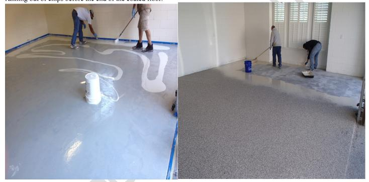
\*This material has a usable pot life of about 30 minutes, work it from the floor, not the bucket. It will overheat if left in the bucket. Pour out on floor in ribbons as soon as it is mixed!
